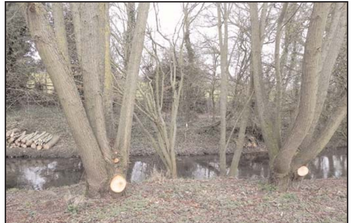
Safety work along Riverside Way.
