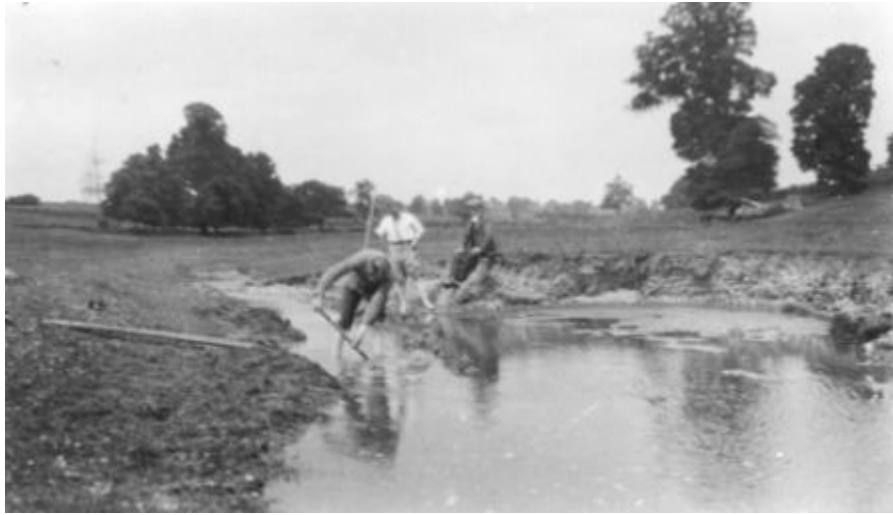
Above: Clearing the river, c1913, Flamstead.
