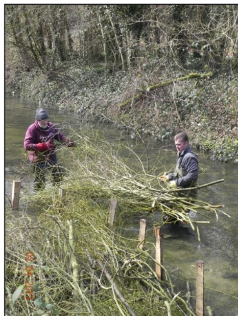
One of the deflectors being installed. [Sue Frearson]
