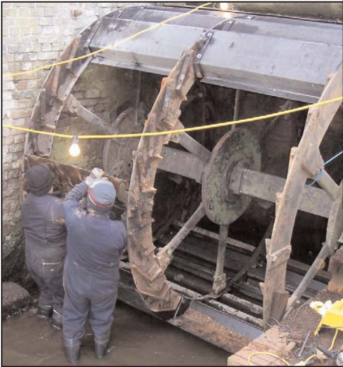
Volunteers cleaning ironwork and fitting new buckets.
